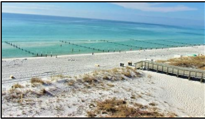
FIRST FIVE SAND GROINS ON OKALOOSA ISLAND
